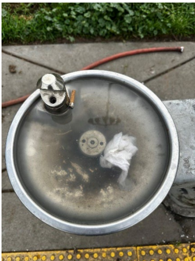
Nonfunctioning and clogged water fountain
