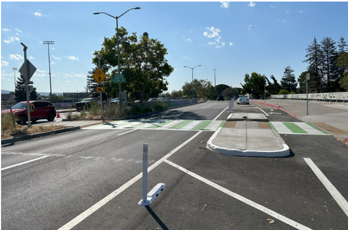
Restriped mid-block crosswalk with concrete islands
