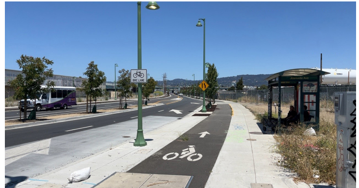
Raised separated bike lane installed on Fruitvale Ave
