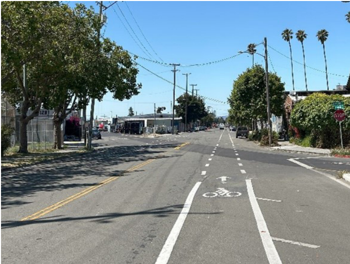
After: Railroad tracks were removed and the bike lane was straightened
