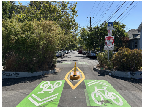
Redesigned bike filter with island and markings
