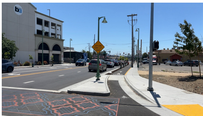
Separated bike lane ramps up at Fruitvale BART
