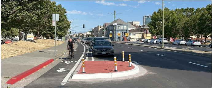
New concrete island and parking protected bike lane on 7th St project rather than a grant-funded capital improvement project. The intent is to strike a balance, providing the most durable and effective bikeway separation at a cost and level of complexity that allows these improvements to be incorporated while delivering the City’s ambitious Five-Year Paving Plan.
