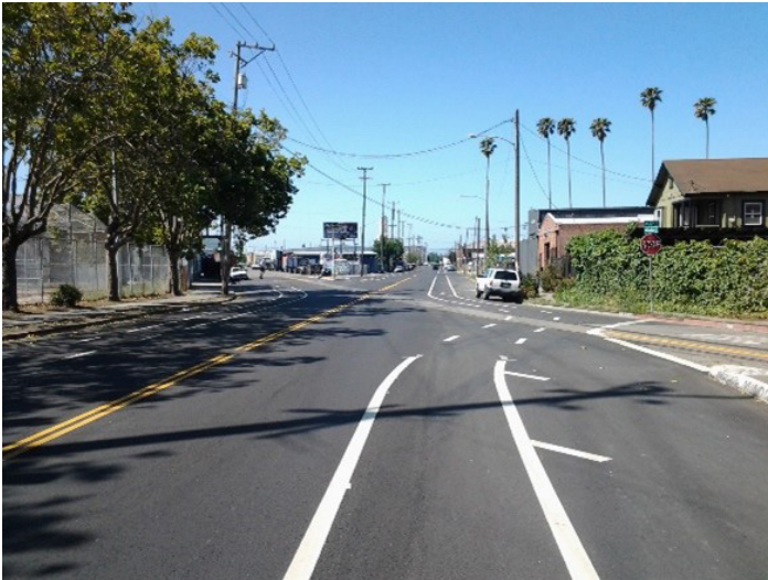
Before: “weave” alignment of the Peralta St bike lane across railroad tracks
