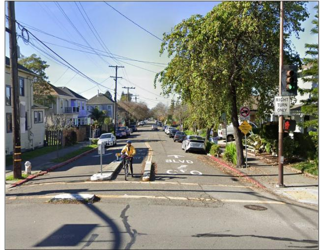
Figure 8: Island cut-through (Channing St, Berkeley)
