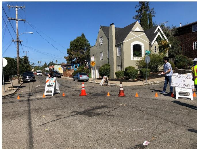
Figure 6. Diagonal diverter made with chalk and cones
