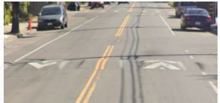
Speed cushion on 38th Ave.
