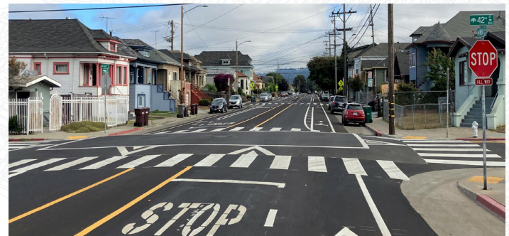
Raised intersection on West St & 42nd St.
