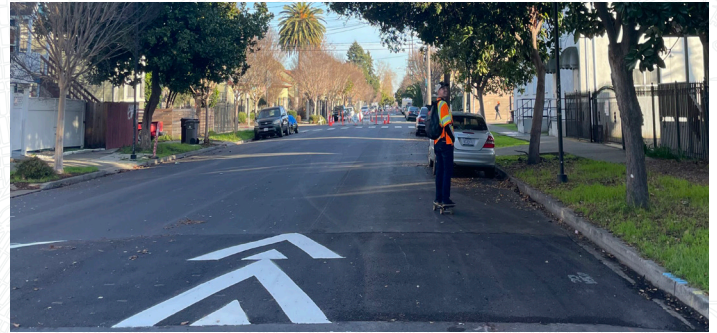
Speed hump on 8th St in West Oakland.
