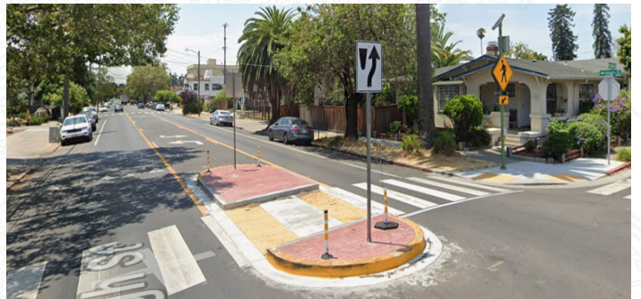
Pedestrian safety island on High St at Suter St.
