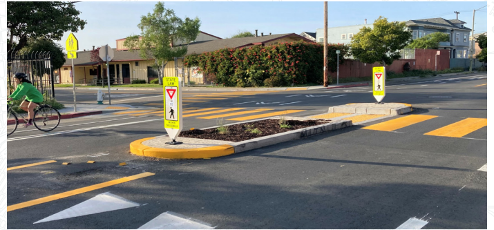
Planted pedestrian safety island on West St at 33rd St.
