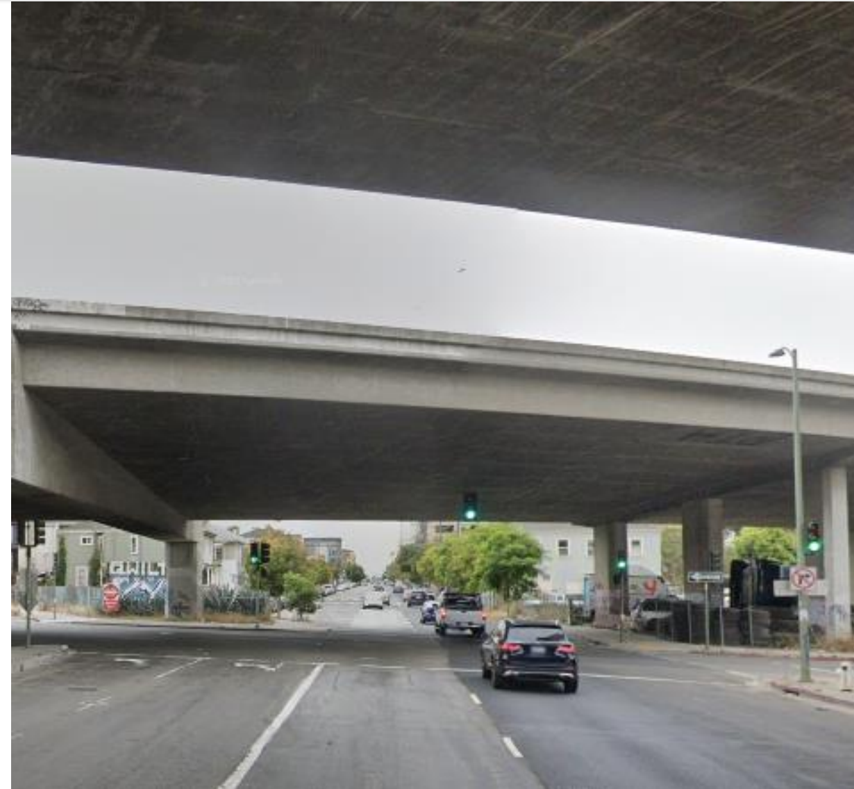
7 th St, under I-980, looking east
