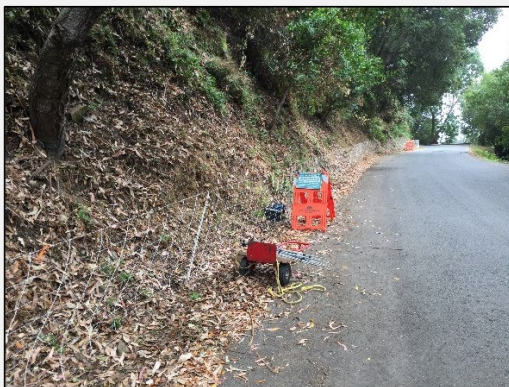
Exhibit 2. Fencing installed along roadway for grazing management.
