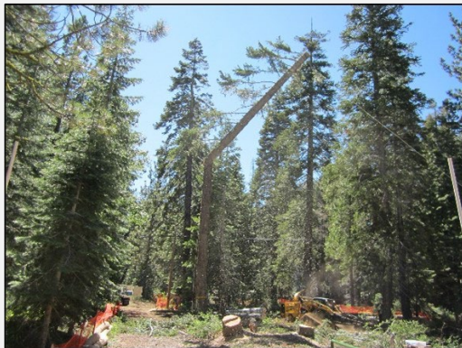
Exhibit 10. Tree being removed in segments.
