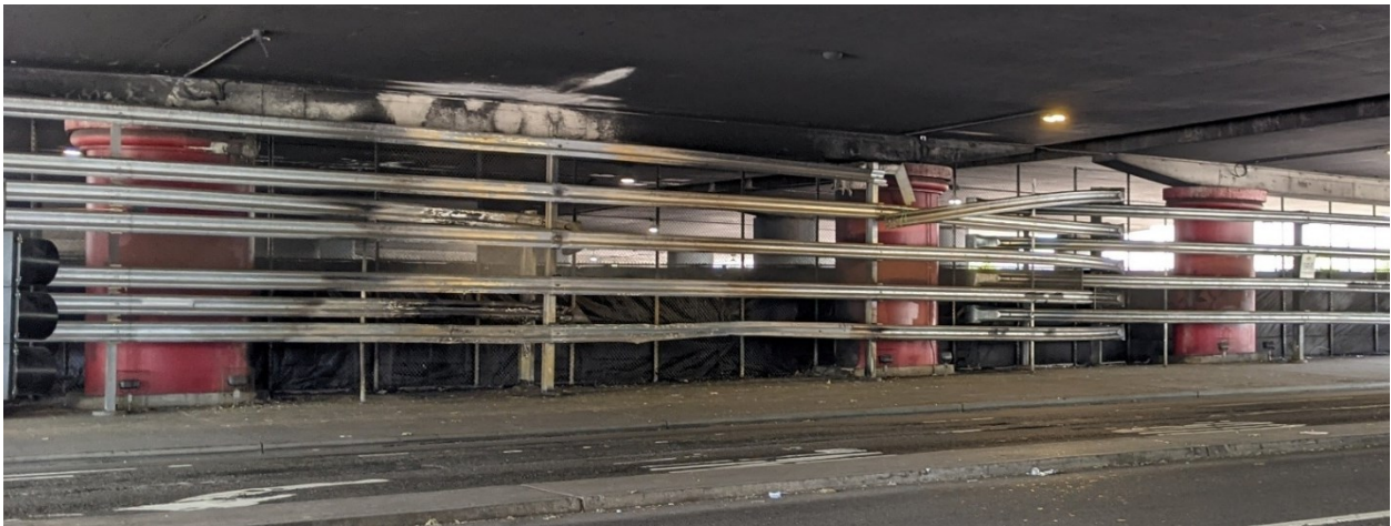
Figure 1. Existing Conditions at Broadway and I-880
