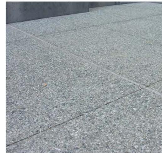
**2. CIP Concrete Paving - Finish 2**
