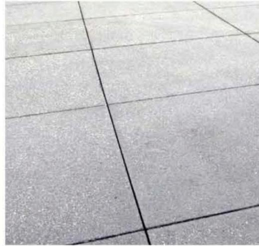
3. CIP Concrete Paving - Finish 3
