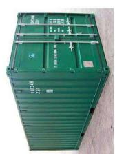
Insulated Intermodal Containers (used as the base of the Cold Storage Structure): ribbed steel, painted to match the Hardi Panel siding on the wood framing above.
