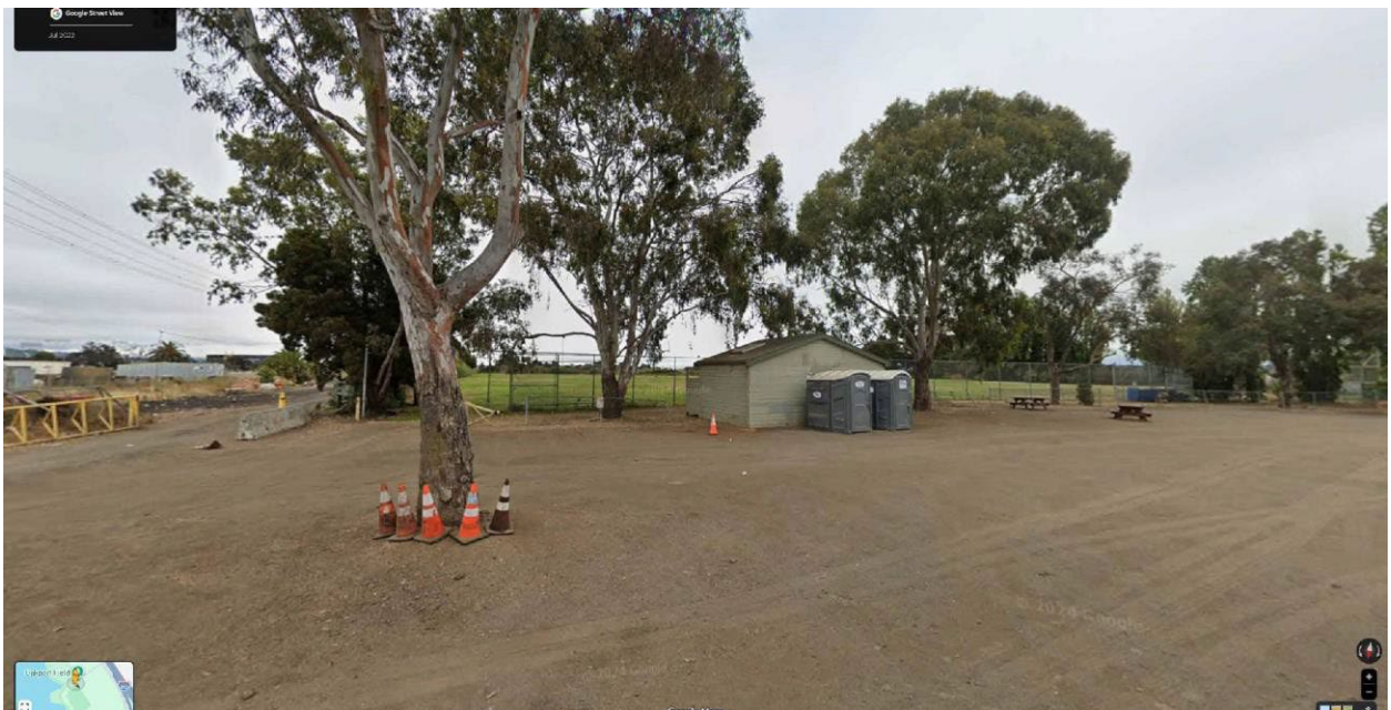
Existing restroom structure and chain-link fencing with fields beyond
