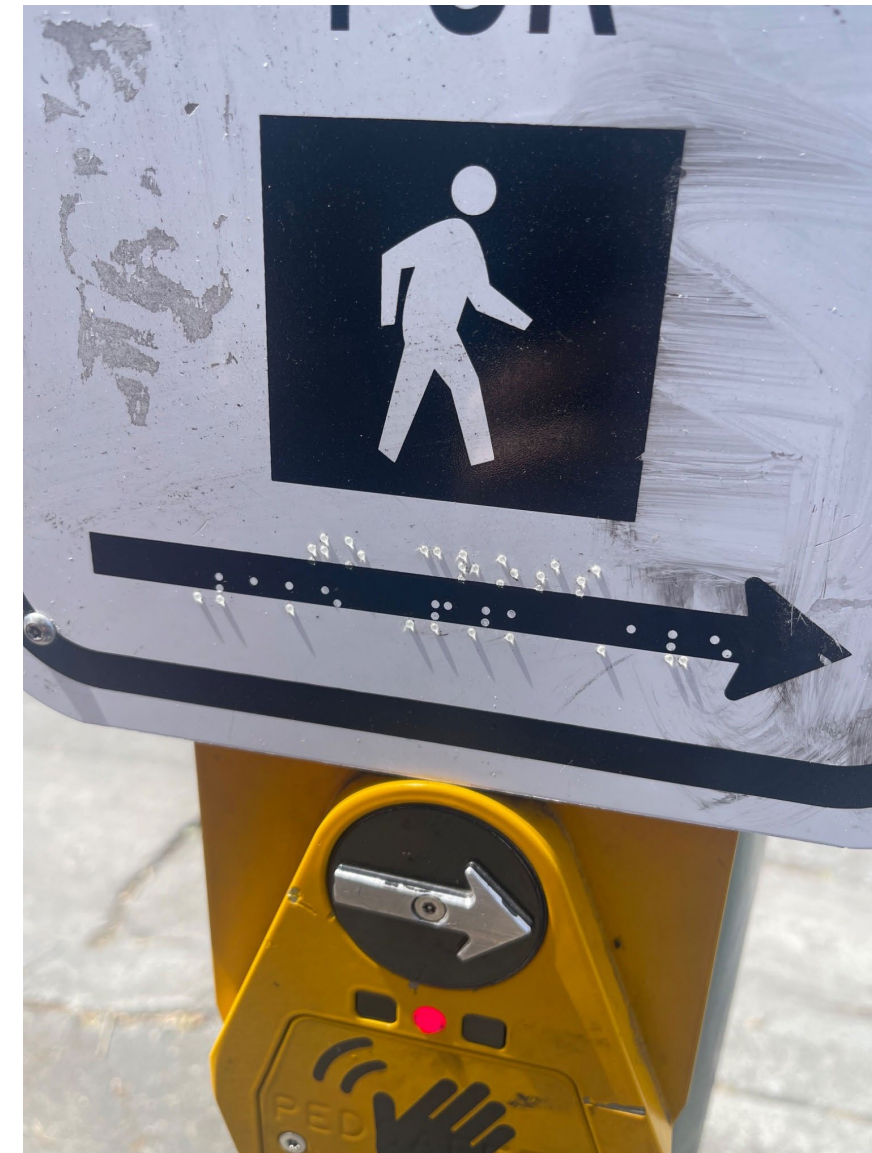
Image shows a pedestrian push button sign-plate, with what looks like braille. The attempt at braille isn't all tactile
