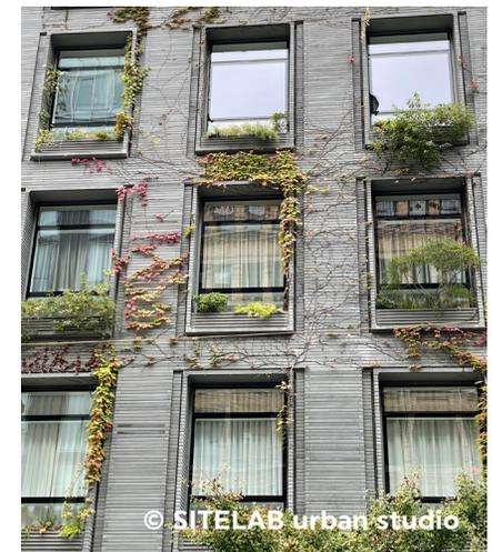
**Figure 2.28:** Examples of enhanced opening depth
