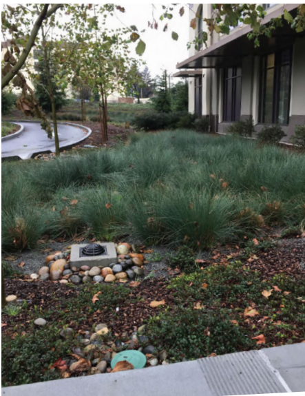
Bioretention: Private Redevelopment, Broadway & 51st St (Oakland GSI Plan)
