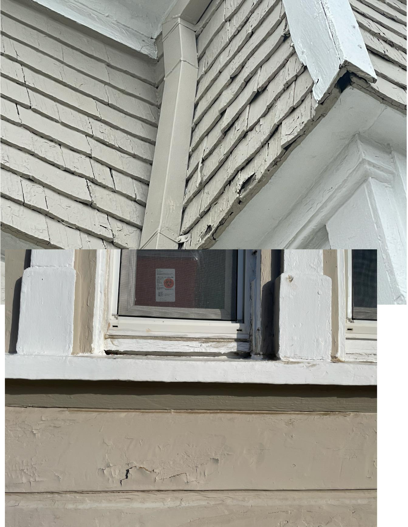
**Work Program Year 9: Paint chipping away to expose raw v-channel siding (below).**
