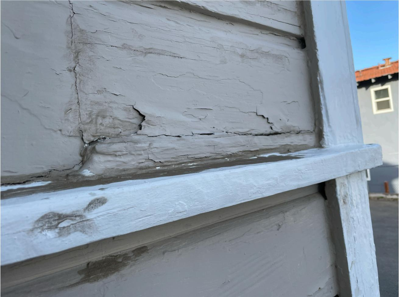
**Work Program Year 9: V-channel siding is mismatched and paint chipping away to expose raw siding.**
