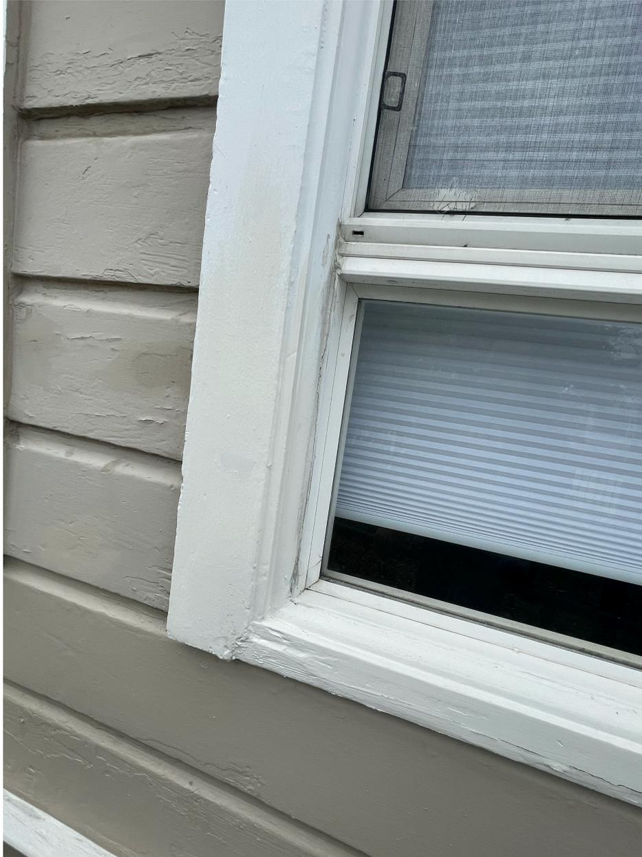
**Work Program Year 9: Trim is poorly fixed, using pieces that don't fit together and expose the fasteners. Evidence of rotten wood that was simply re-painted (see deeply grooved horizontal grain under paint at base of window trim). Spurious plaque installed by previous owner.**
