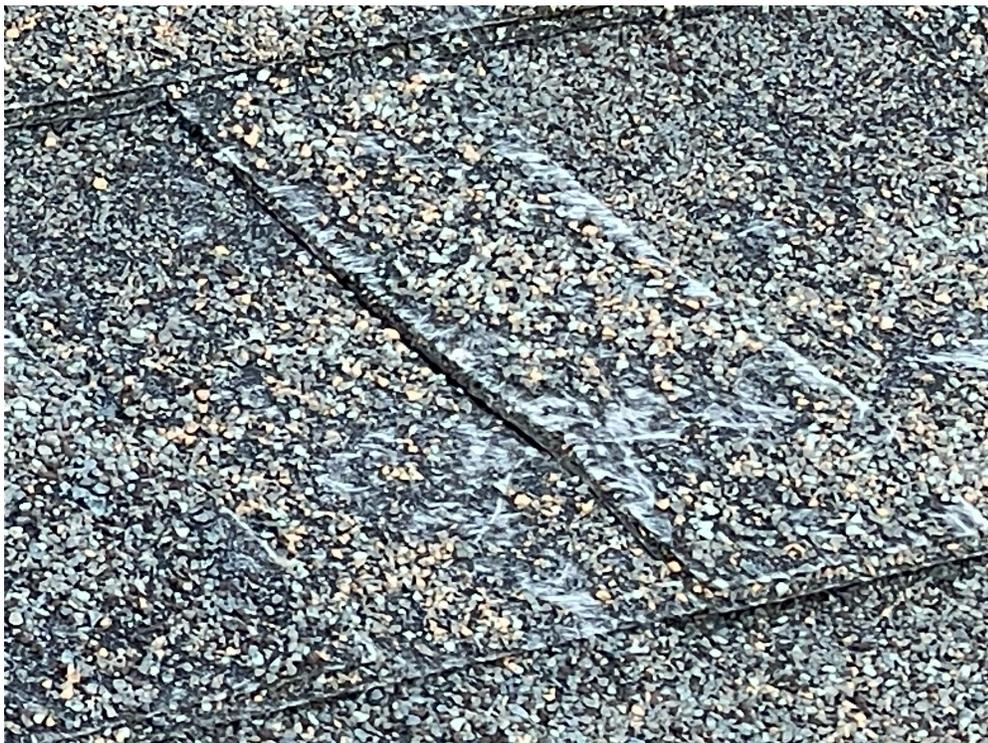
**Closeup of shingle detail shows the material worn down to the fibers.**
