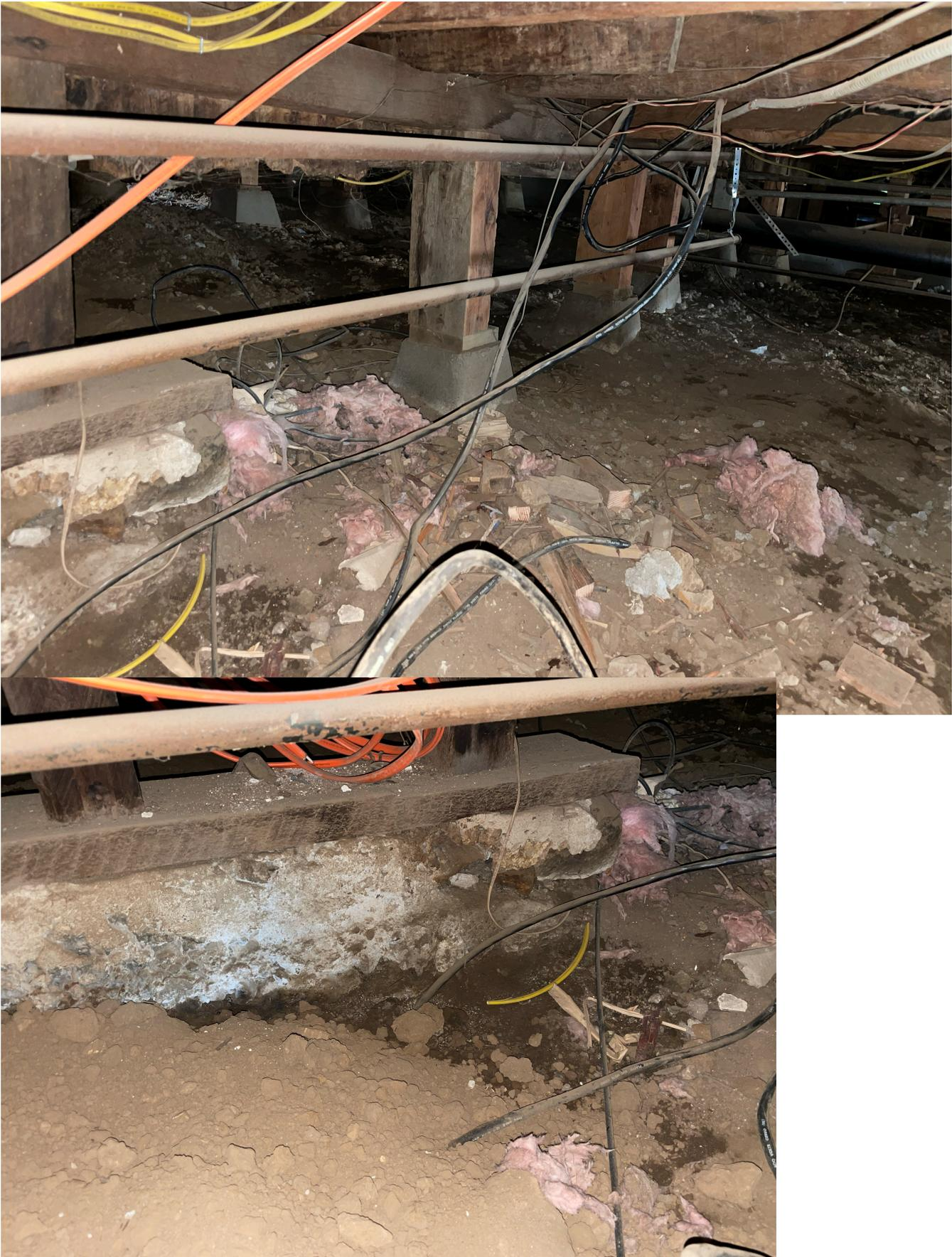
**Work Program Years 2 & 3: Capped foundation using loose rock rubble as fill and unsettled cure (trapped air bubbles when concrete was wet) yielding inconsistent support.**
