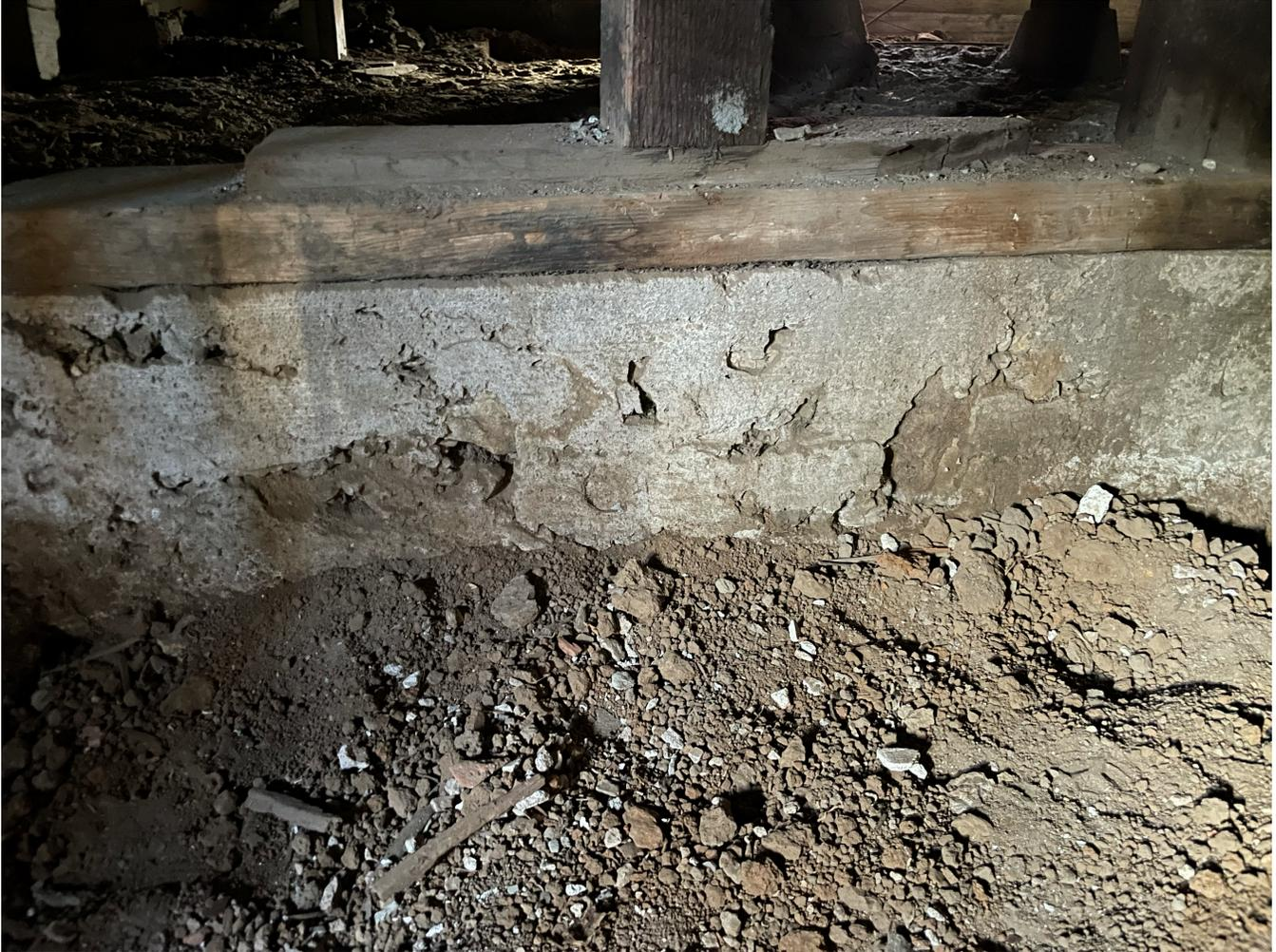
**Work Program Year 4: Evidence of pest infestation in foundation framing and floor joists.**
