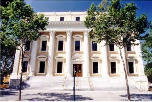
The courthouse, listed on the National Register of Historic Places, was constructed in 1866, partially rebuilt after a 1931 fire and damaged during the Loma Prieta Earthquake. Unreinforced masonry walls and a steel frame provide support for a concrete roof and floors.
