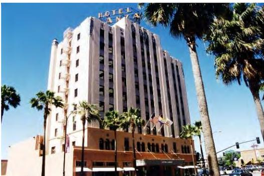
This project required the rehabilitation and seismic retrofit of an 85,000 sf 11-story historically significant art deco concrete structure.
