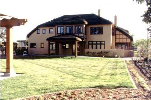
The Ainsley House is a two-story wood frame structure built in the 1920s, which was relocated along with its detached two-story garage from its original site to a reinforced concrete foundation/basement several miles away. Structural work on the project began with the preparation of a preliminary seismic analysis and report for use in estimating restoration costs and feasibility.
