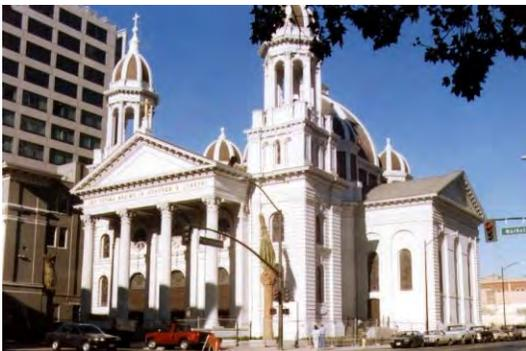
Biggs Cardosa performed the seismic retrofit and rehabilitation of St. Joseph's Cathedral, one of the most culturally and architecturally significant landmarks in downtown San Jose. The structure was constructed in the late 1800s and features 45-foot tall unreinforced masonry walls, timber roof framing, and three domes supported on timber trusses.
