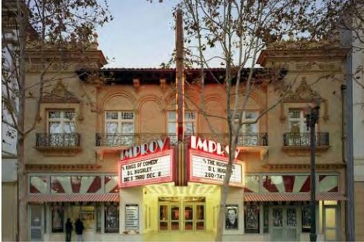
This historic theatre was built in 1903 and is constructed of 40-foot tall un-reinforced masonry walls (URM). The roof consists of a 70-foot long wood truss system. The front half of the building has a wood framed second floor and balcony.
