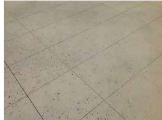
PEDESTRIAN PAVING - INTEGRAL COLOR CONCRETE WITH ROCK SALT
