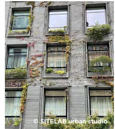
**Figure 2.28:** Examples of enhanced opening depth
