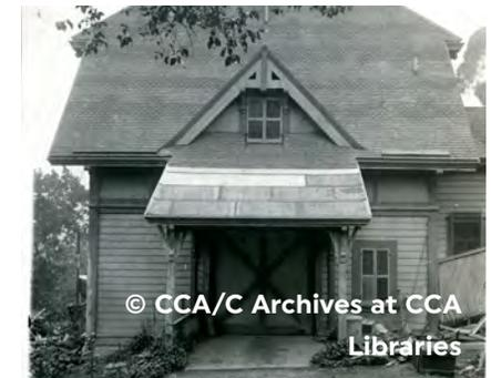
**Figure 2.7:** Carriage House original opening on east facade
