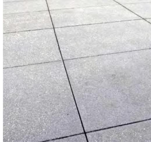
3. CIP Concrete Paving - Finish 3
