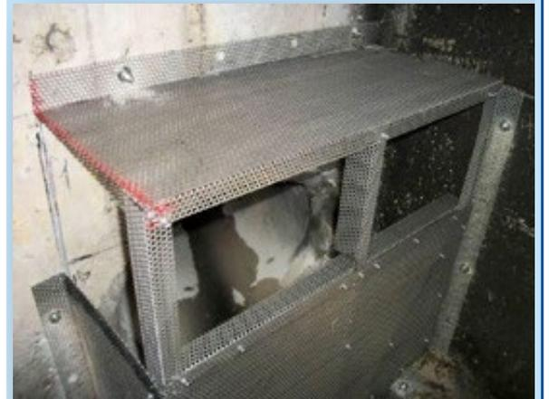
*Inlet Based Full Trash Capture Device*
