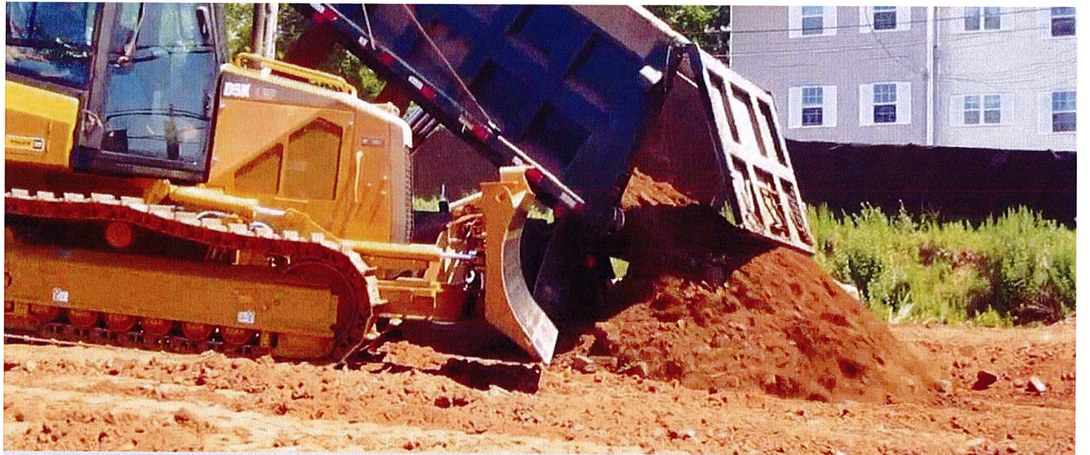
13 FILL AND GRADING
