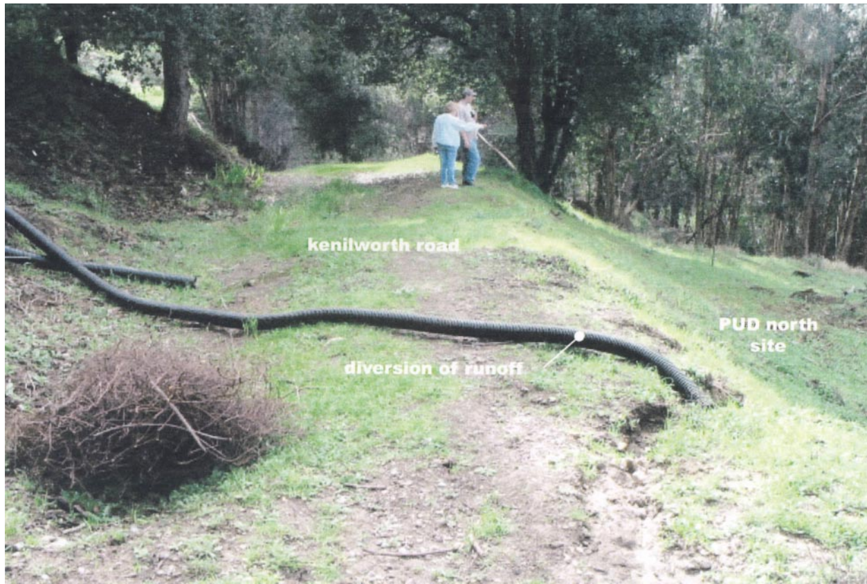
Stormwater concentration and diversion across Kenilworth Road to PUD North Site from nearby upslope properties.
