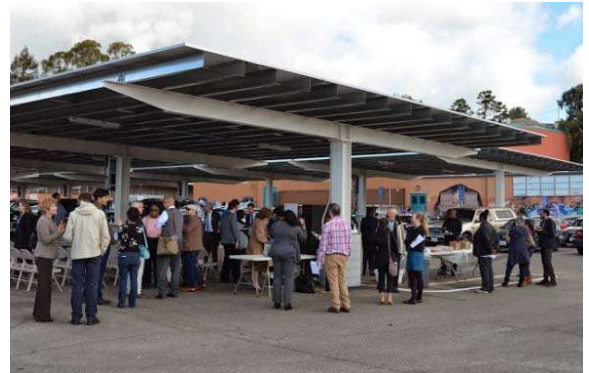
Parking lot photovoltaic array at Castlemont High School – Courtesy of OUSD
