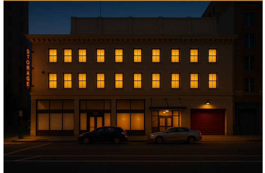
Self Storage on Second & Third Stories
