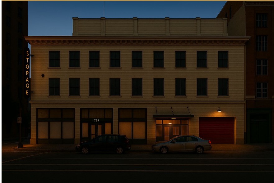
Office on Second & Third Stories
