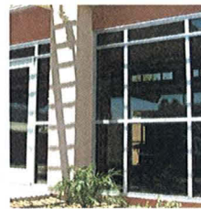
4 ALUMINUM STOREFRONT - ANODIZED W/ CLEAR GLAZING
