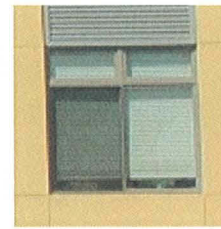
5 FIBERGLASS/ VINYL WINDOW - PEBBLE GRAY W/ CLEAR GLAZING
