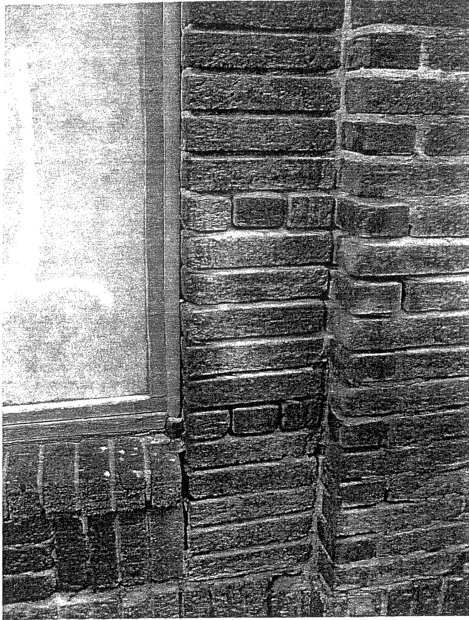
DETAIL - POOR QUALITY MORTAR JOINTS
