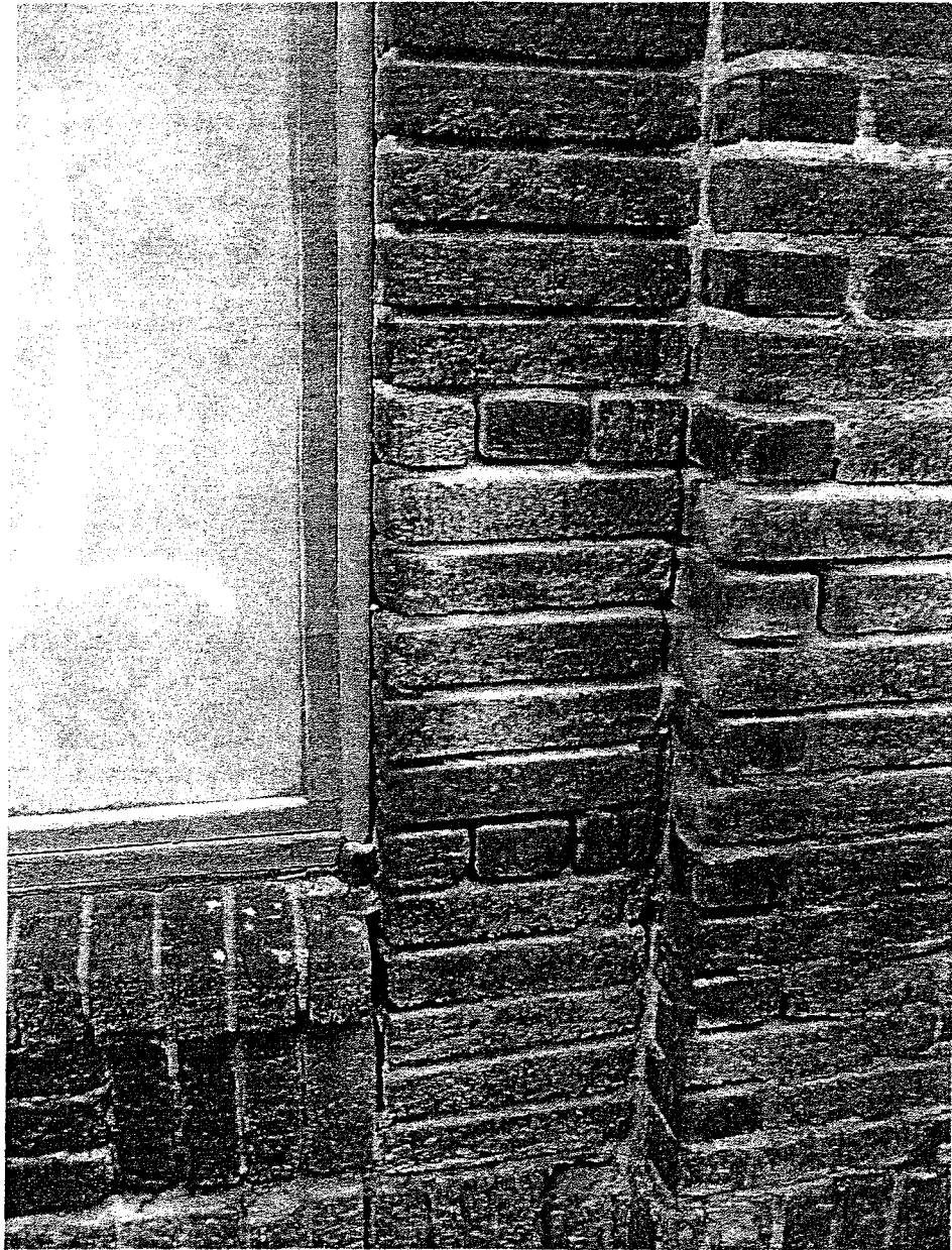
DETAIL - POOR QUALITY MORTAR JOINTS
