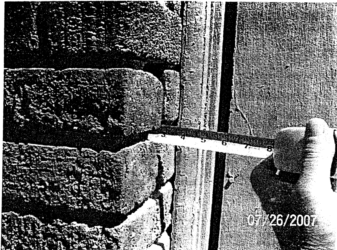
DETAIL - POOR QUALITY MORTAR JOINTS
