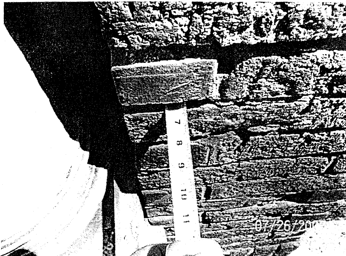
DETAIL - POOR QUALITY MORTAR JOINTS
