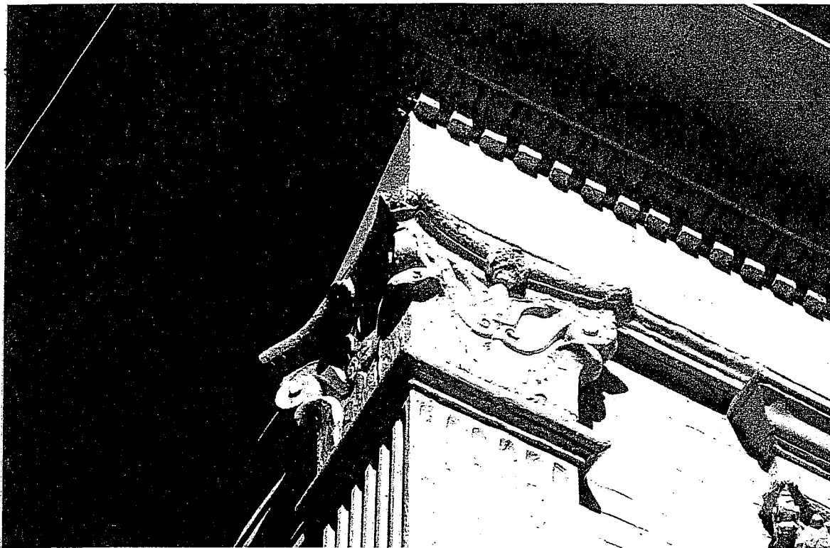
Faux corner column + cap, dentil moulding Work Program # 2,3
