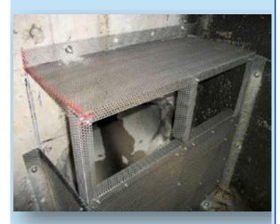
Inlet Based Full Trash Capture Device
