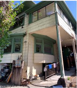
Right side of house – asbestos siding, original vs aluminum sash
