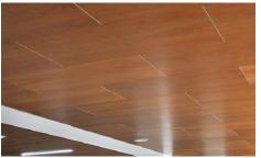
Wood-like exterior soffit finish
