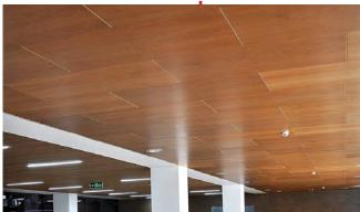
Wood-like exterior soffit finish
