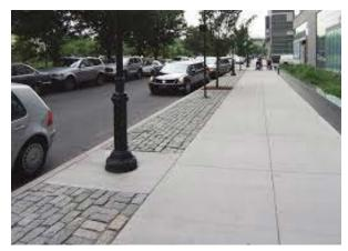
Figure 26: Special Paving between Tree Wells
