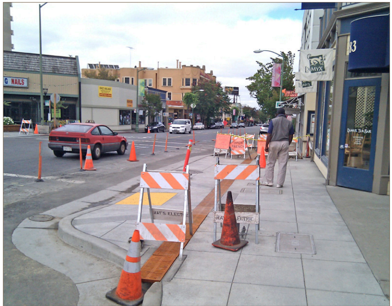
Figure A-4: Sidewalk Bulb-Out Under Construction on Piedmont Avenue, Oakland (Source: Eric Fischer (used under Creative Commons license: http://creativecommons.org/licenses/by/2.0/ ))
