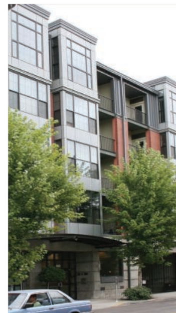
Guideline 6.2: The metallic exterior framing of these windows provide depth to the façade.
