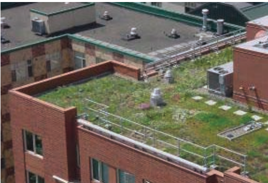
Guideline 6.4: Green roofs filter stormwater
