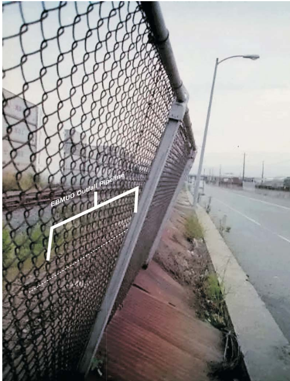
Geologic and seismic damage along the northern boundary of Burma Road in the Gateway development area. To the left is a fence and sidewalk, demonstrating that substantial settlement has occurred in the area. The top of the East Bay Municipal Utility District outfall pipeline is to the left of the fence. This pile-supported structure has remained stable, while surrounding fill has not.
