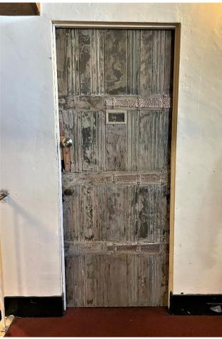
Figure 11. Door with decorative strap hinges, northeast side of mezzanine.
