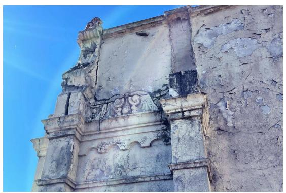
Figure 4. Plaster decorative elements at parapet, view southwest.
